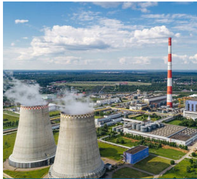
Athena Power Plant, Chattisgarh
