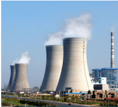
Khurja Power Plant, Khurja
